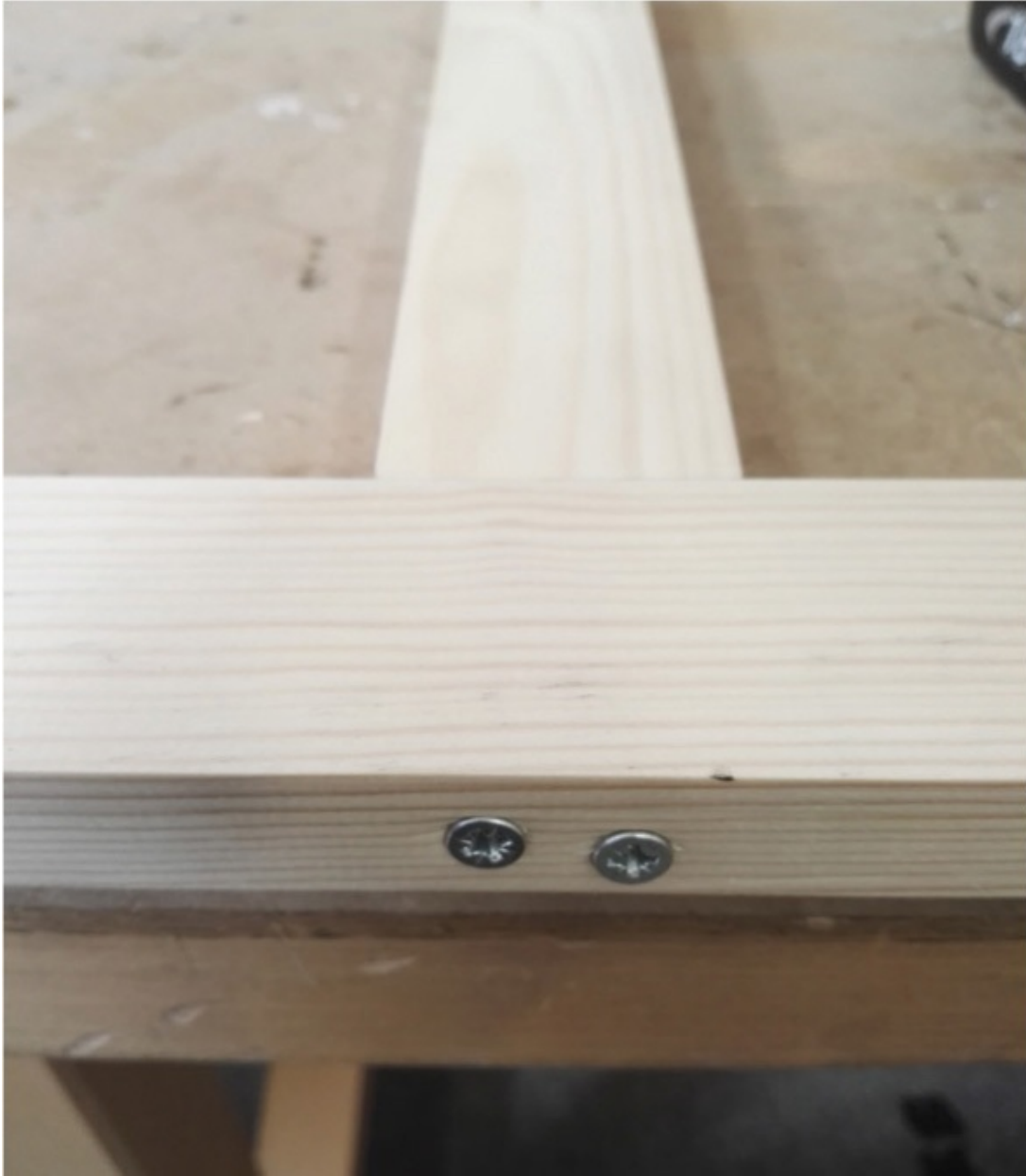
Cross bars are inserted into the middle of the frame away from the top edge. These were butt jointed and secured by drilling through the strainer bars into the cross bar and then screwed together.
