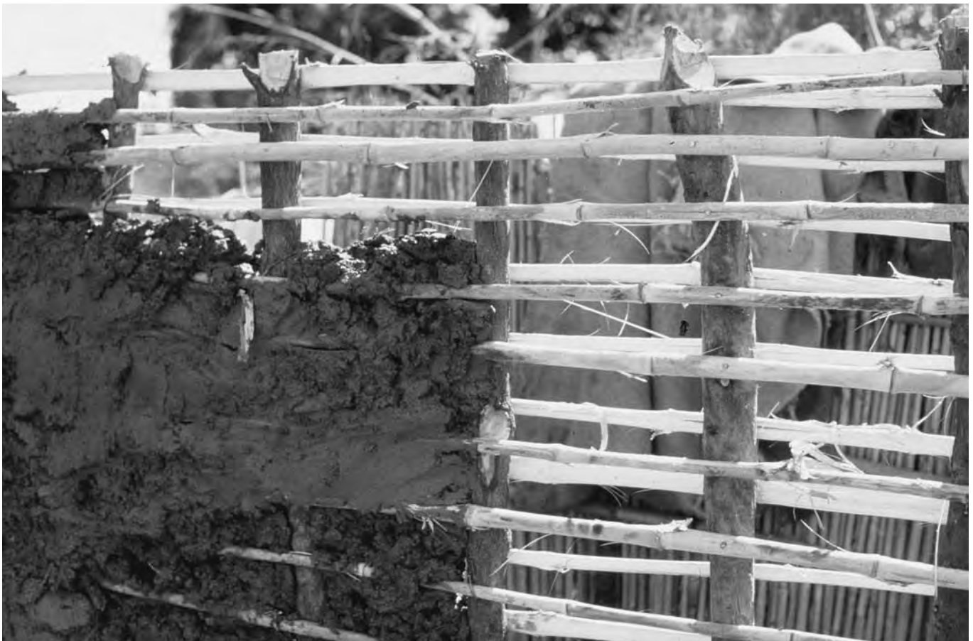
Wattle framework being filled with red mud, a construction technique used in ancient times, from Zambia (© Board of Regents of the University of Wisconsin System)
