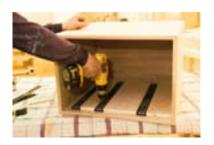
Using spacers to position the drawer slides eliminates one of the leading causes of poor-fitting drawers: inconsistent spacing of slides. Before putting in the spacers, be sure to brush out any sawdust or woodchips that may have accumulated inside the cabinet. A 1/16" discrepancy at this point could cause an annoying misalignment that you'll have to backtrack to correct later on.
