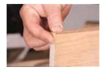
To trim the edge, start by carefully bending over the ends until the
