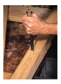
Now square up the edges of the mortise using a mortise chisel and a small mallet (step 6).
